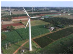
Generating power: A wind farm at Gudimgalam in Tiruppur district of Tamil Nadu is 30% operational
